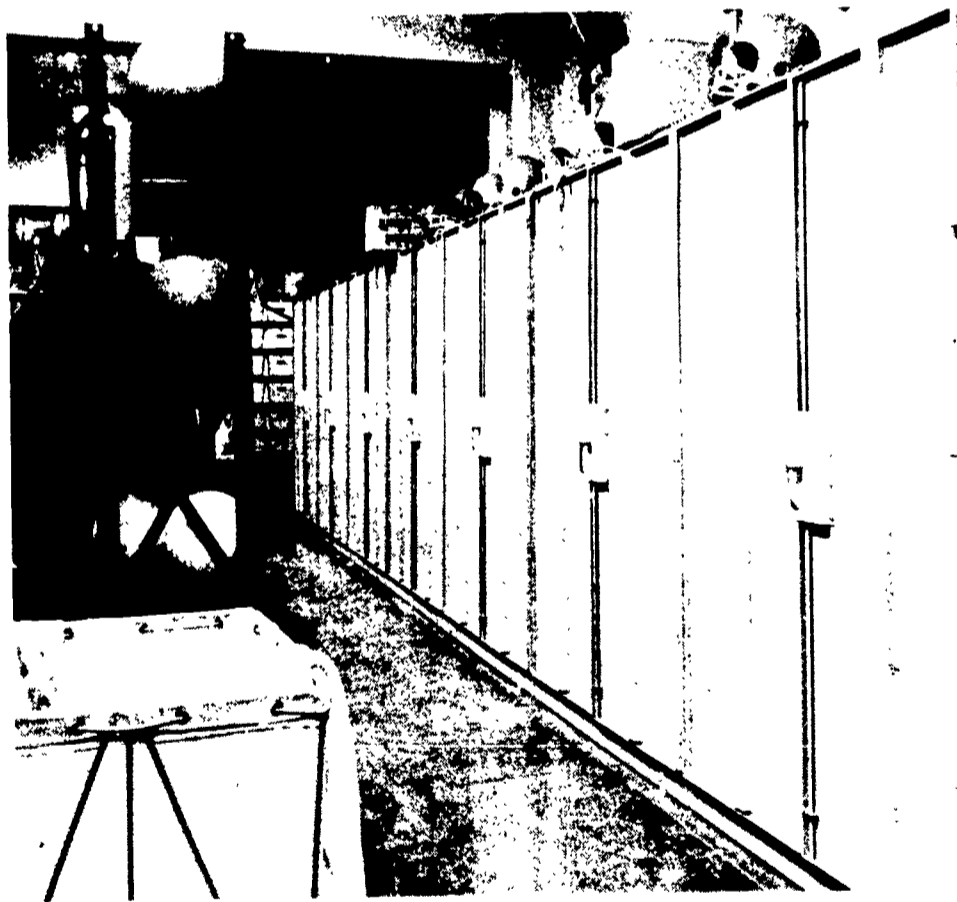
"Rear access doors" - each pair of doors opens 30 box gym lockers.
